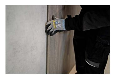
At 7.8 mm thick, RESOPAL SpaStyling Boards are a lightweight, excellent solution for new and renovated wet rooms. They can be installed on-site in very clean conditions with minimal downtime.
