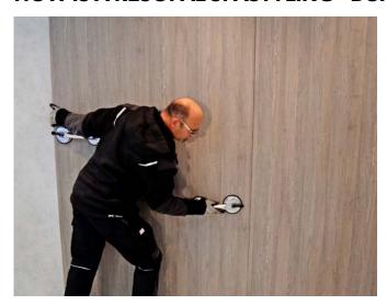
RESOPAL SpaStyling Boards can be treated and machined with standard tools directly on site, just like standard wood materials. The RESOPAL SpaStyling Board can be adhered directly to existing tiles or other substrates in new construction and renovation projects. The quick, easy and clean installation ensures little dirt and little downtime.
